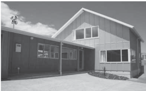
FIGURE 4.1: Main approach exterior view
